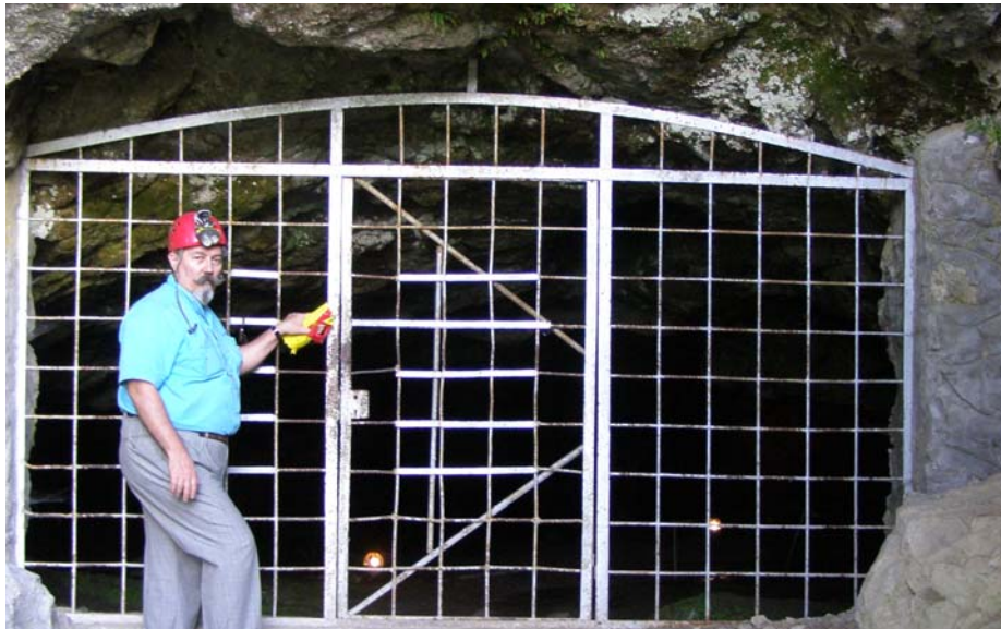
Fig. 11. Southern entrance with an actually unsuitable gate (15 × 15 cm net of lattice) not allowing bat flying access.
